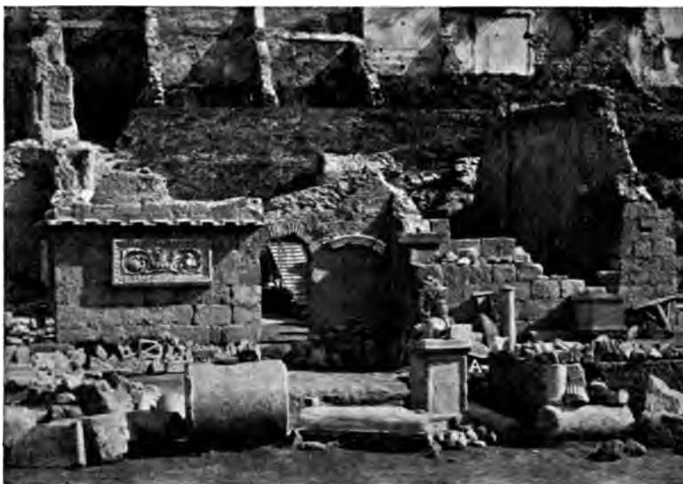
Remains of a mediæval building occupying part of the Basilica Æmilia, where an important fragment of the Fasti has been found, used as a threshold at the point marked A.
